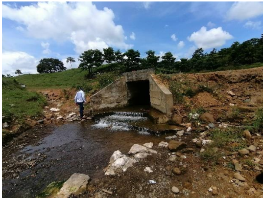
Vista box culvert.
