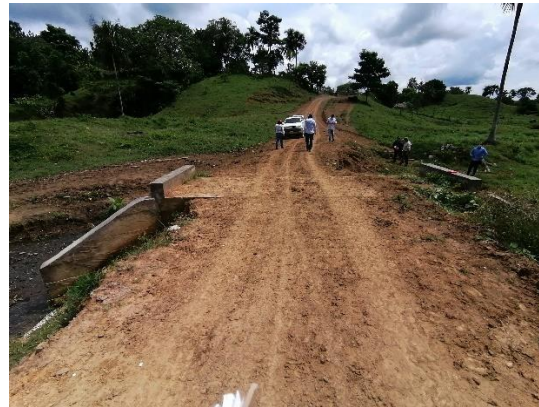
Detalle general box culvert.
